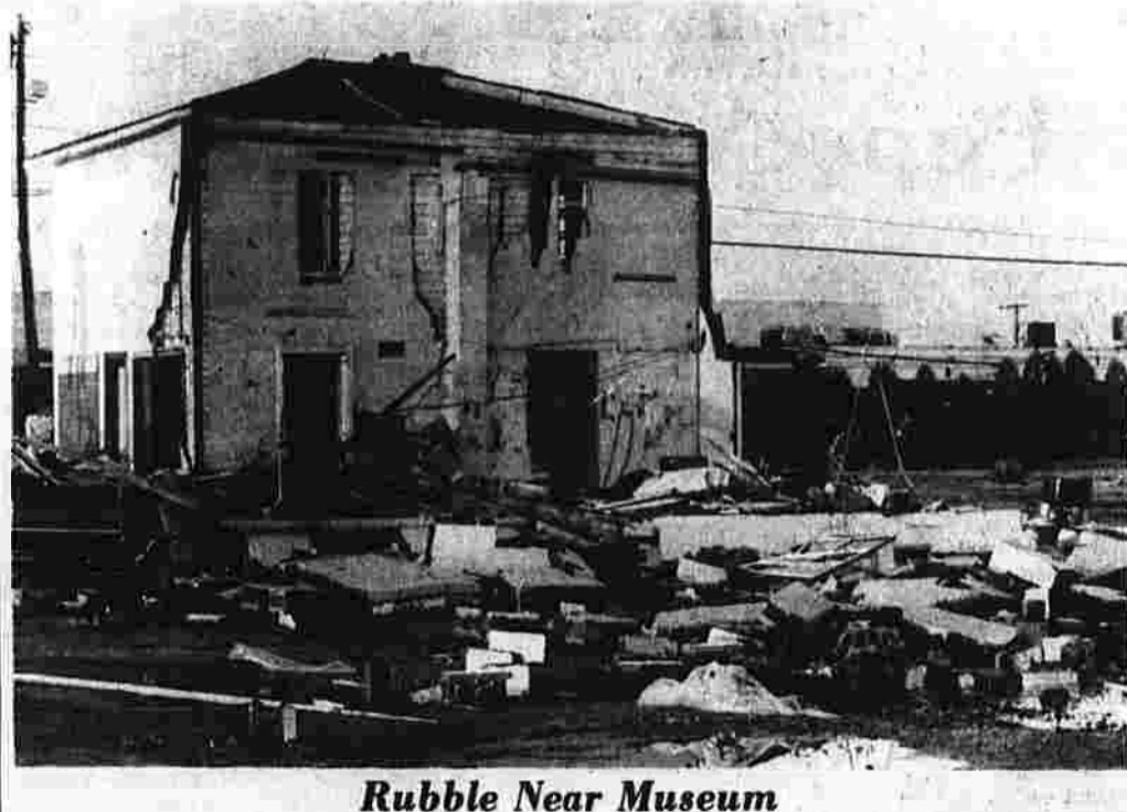
Rubble near Museum. One section of the building was torn away during the freak storm. (Herald photo by Adamson)
