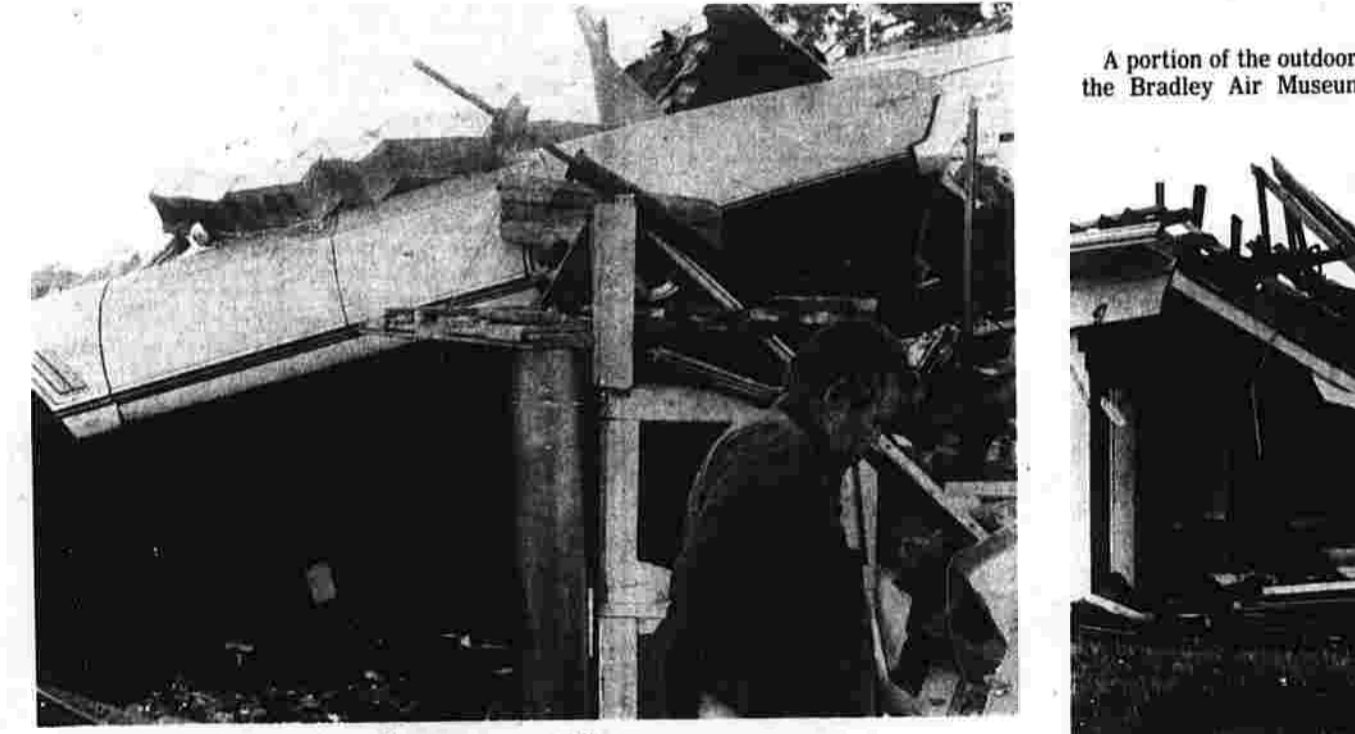
Damage at Garage
