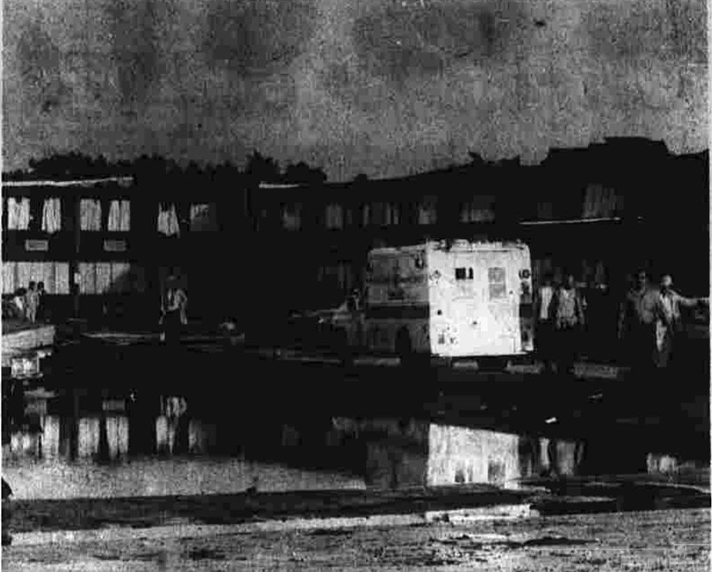
An ambulance stands by late Wednesday afternoon at the Koala Inn, Route 75, Windsor Locks, to evacuate injured persons from the hotel. The hotel was heavily damaged by the storm which cut a swath down Route 75 from the Bradley Air Museum. (Herald photo by Adamson)
